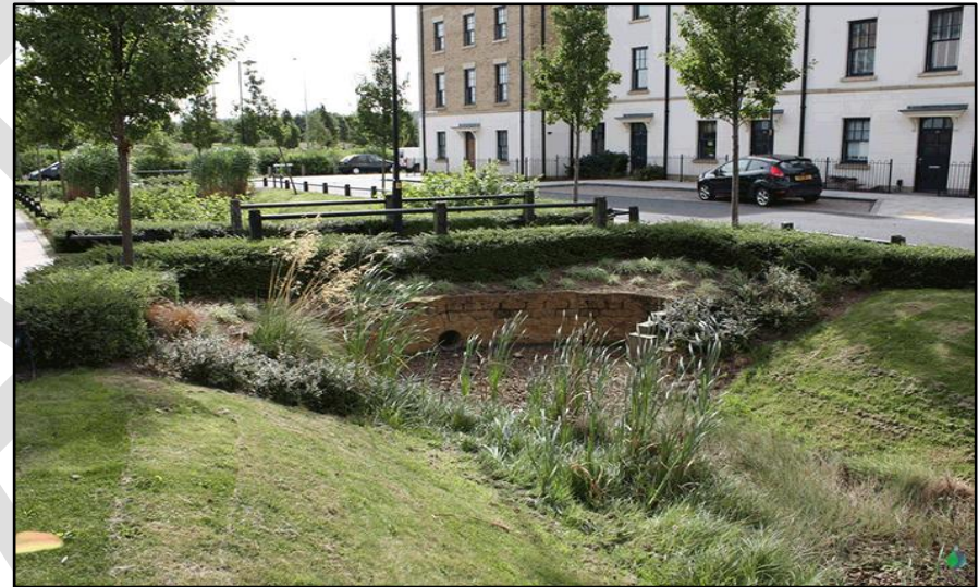
Sustainable Drainage System retrofitted in Mansfield
